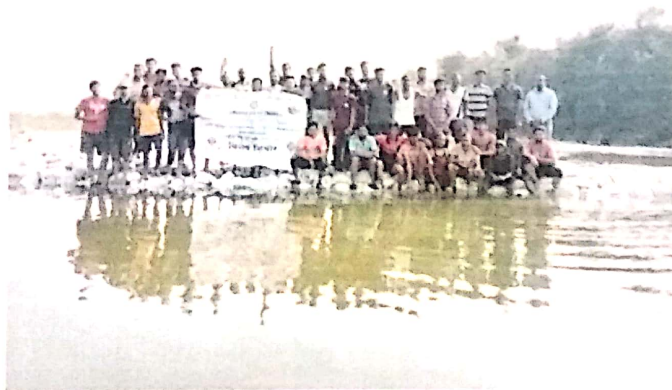
Completion of Bandhara at Bhima River
