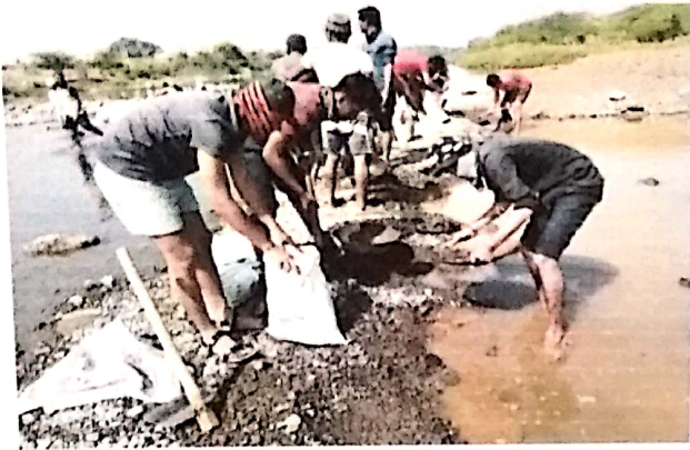
Construction of Bandhara at Bhima River
