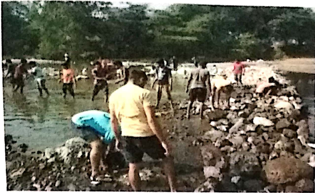
Construction of Bandhara at Bhima River
