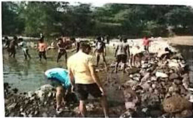
Construction of Bandhara at Bhima River
