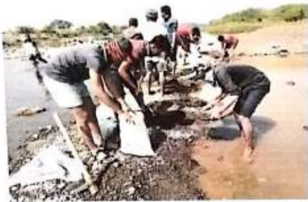
Construction of Bandhara at Bhima River
