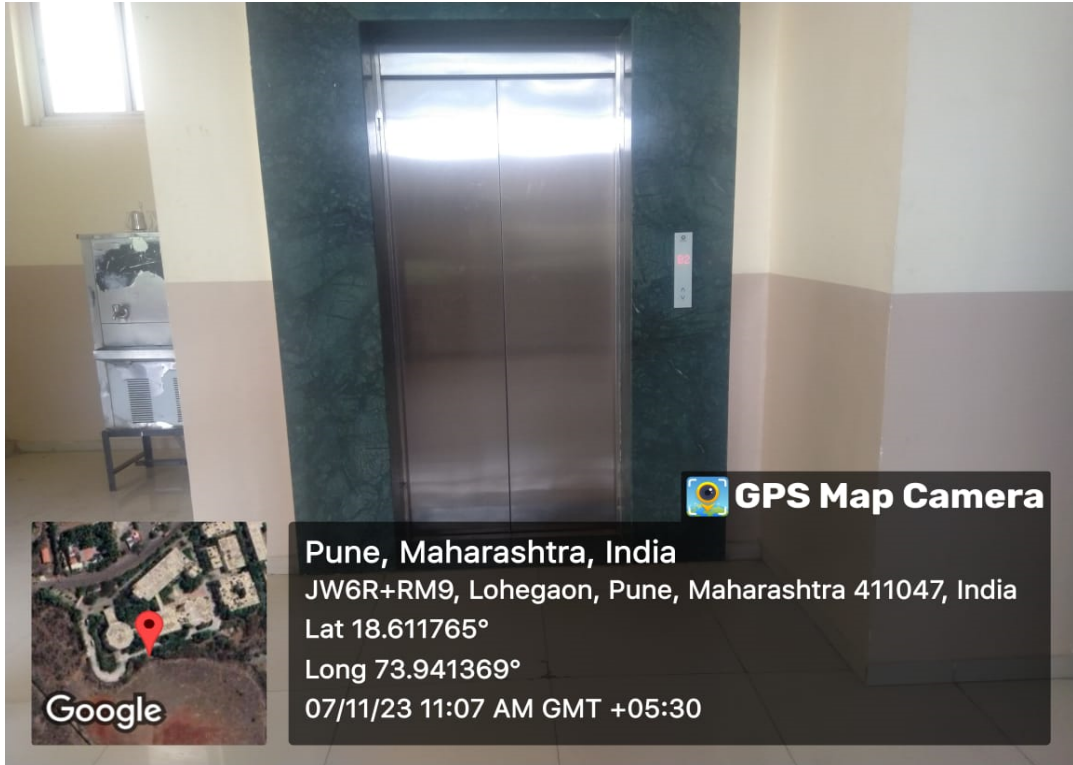
1. Geotagged_Main Building Lift 1
