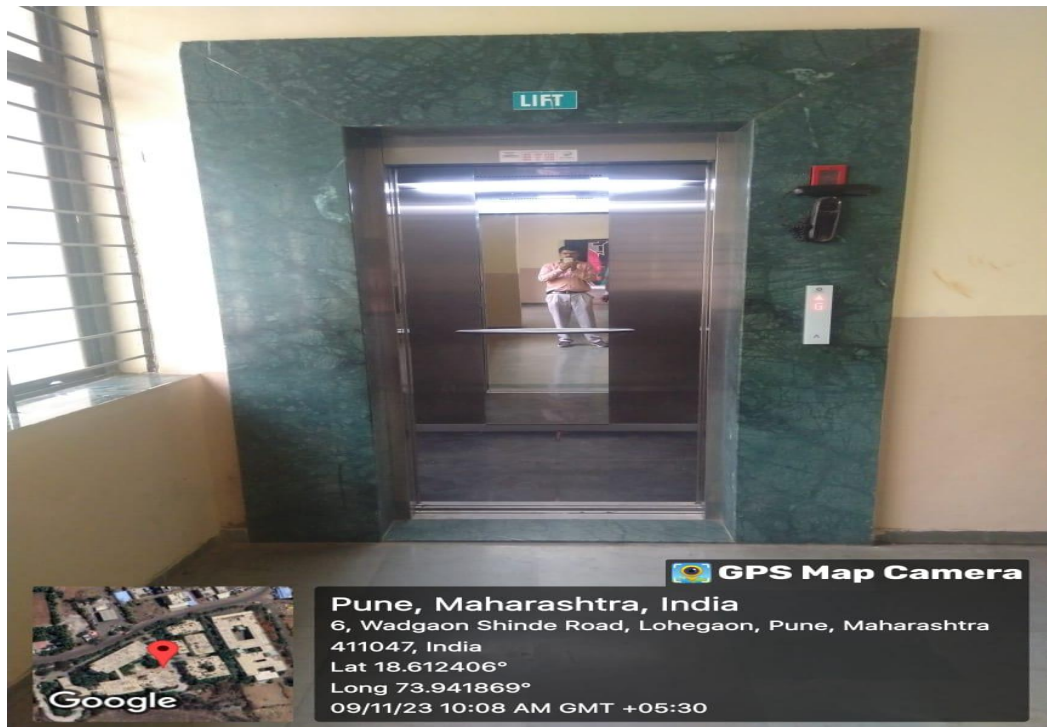
2. Geotagged_Main Building Lift 2
